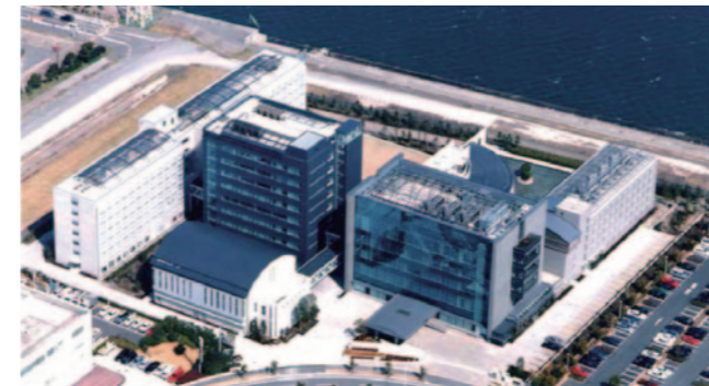
URAYASU Center, Research and Training Institute of the Ministry of Justice. Housing the Research Department and Training Facilities
