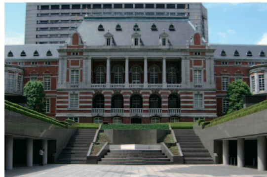
The red brick building seen from the sunken plaza
