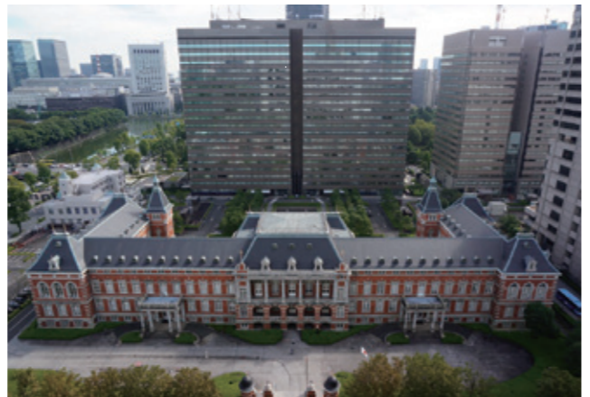
Red-Brick Building and Central Government Office No.6-A
