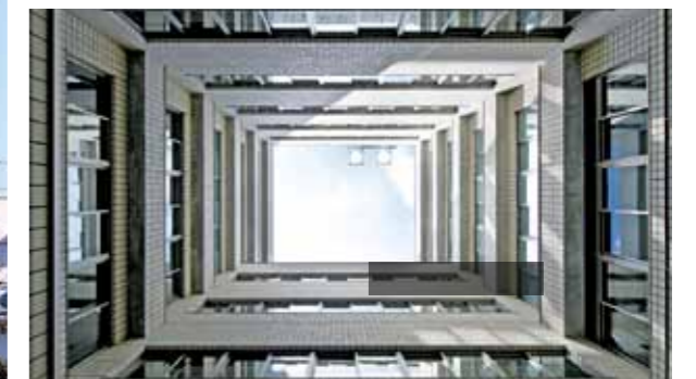
Kofu Ministry of Justice Office Complex
