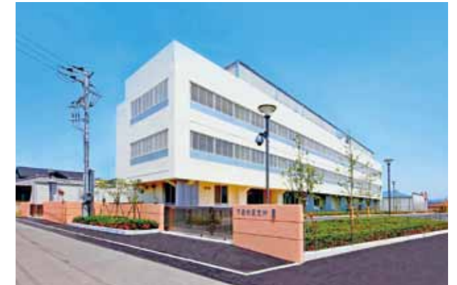
Renovation of the Shimotsuma Detention House (constructed in 1964) [2018]
