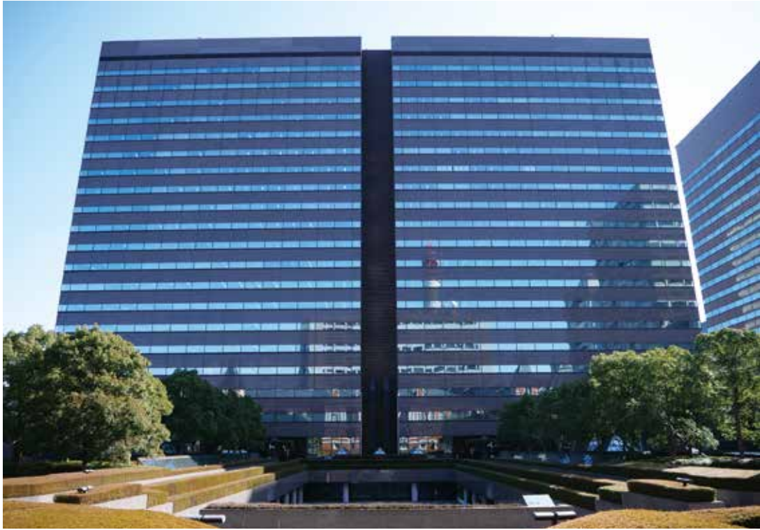
Central Gov't Bldg. No.6
