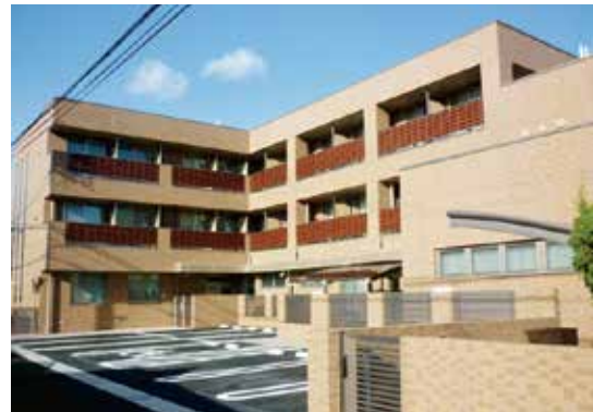
Exterior of an Offender Rehabilitation Facility
