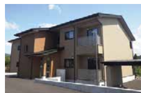
Official residence of Konan juvenile school (Introduction of the wooden structure (CLT structure))
